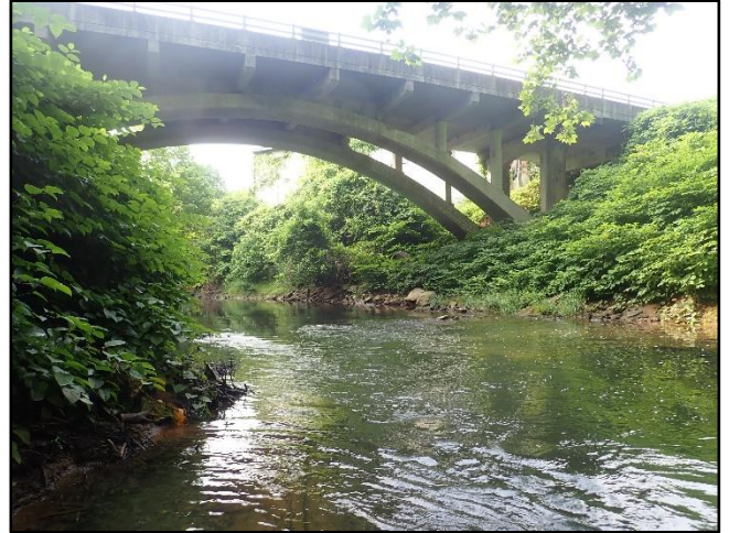
PR-10, Looking upstream
