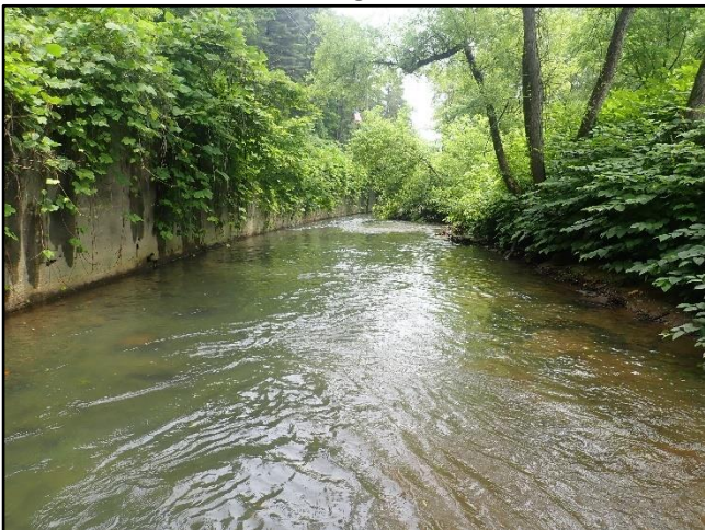
PR-35, Looking downstream
