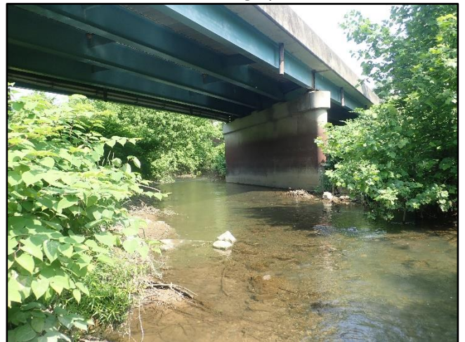
PR-27, Looking upstream
